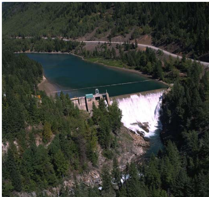
Photo courtesy of BC Hydro
